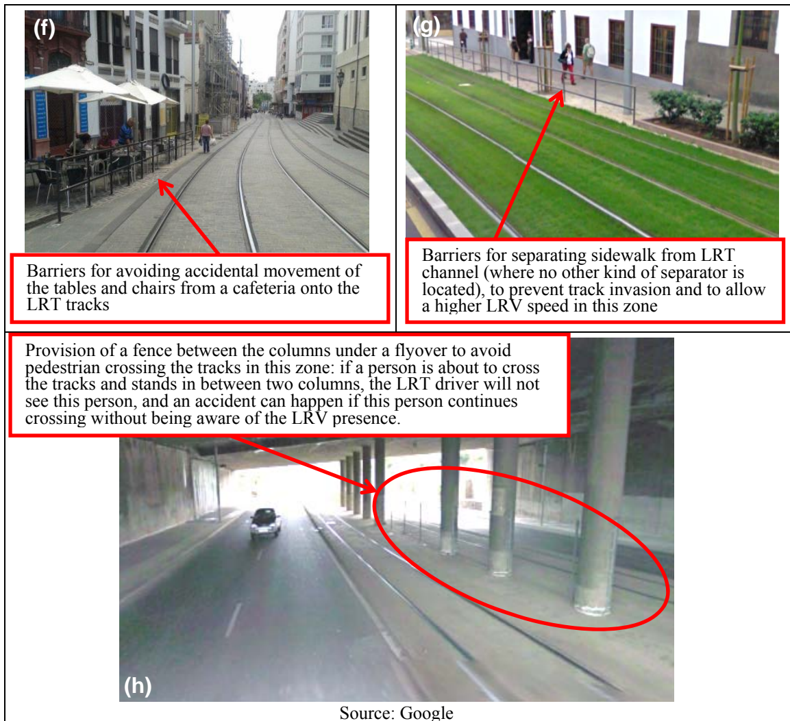
FIGURE 9 LRT channel differentiation and protection by means of pavement, marks, fences and barriers. a,b&c) Pavement treatment to avoid LRT tracks trespassing by road vehicle drivers in Dublin; d) Pavement treatment of a segregated channel in Dublin; e) Demarcation of swept path on shared channel in Dublin; f&g) Barriers for avoiding invasion in Tenerife; h) Fences for avoiding pedestrian crossing under a flyover in Tenerife.
