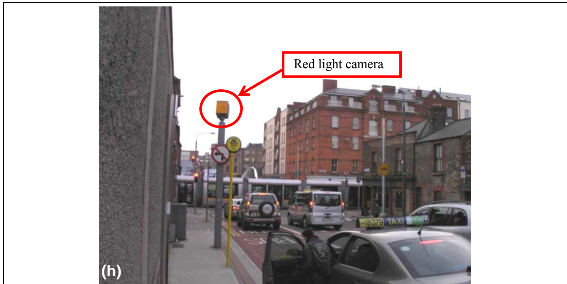
FIGURE 8 Innovative solutions at intersections. a,b&c) LED lights embedded in the pavement in Barcelona; d&e) Flashing red road studs in Dublin; f&g) “See-through” problem with louver solution in Dublin; h) Red light camera in Dublin.
