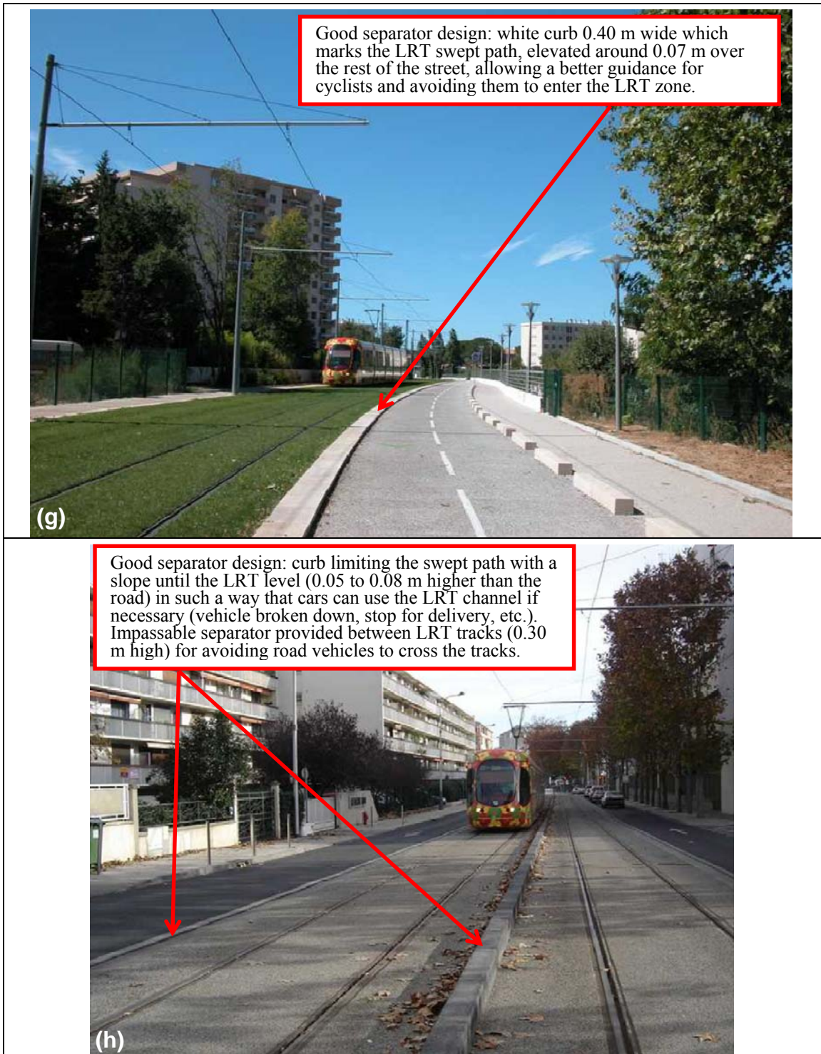
FIGURE 4 LRT separators on segregated channels. a) Parking forbidden along the separator in Tenerife; b,c,d&e) Green separators in Porto; f) Sidewalk-alike separator in Montpellier; g) Curb separator in Montpellier; h) Curb separator between both LRT directions in Montpellier.
