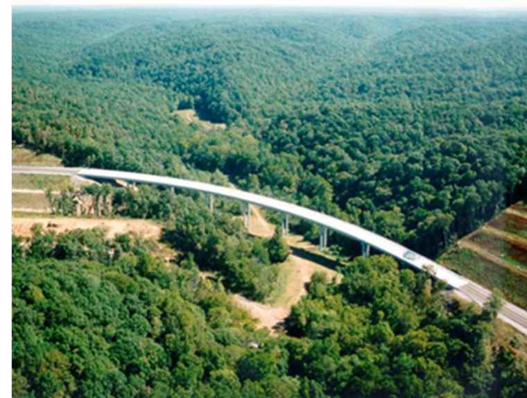
State Route 50 - Bridge over Happy Hollow Creek – Tennessee – 1175feet long (358 m)
