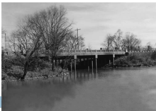
SR 7 Teens Run Bridge at Eureka in southeastern Ohio – 1938 – Source “Integral & Semi-Integral Bridges” Martin P Burke Jr
