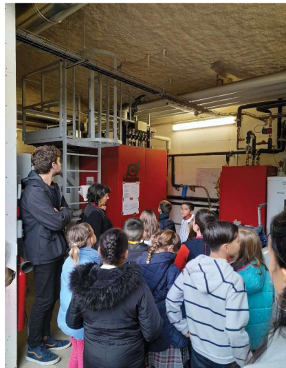
Visite chaufferie (Rillieux)
