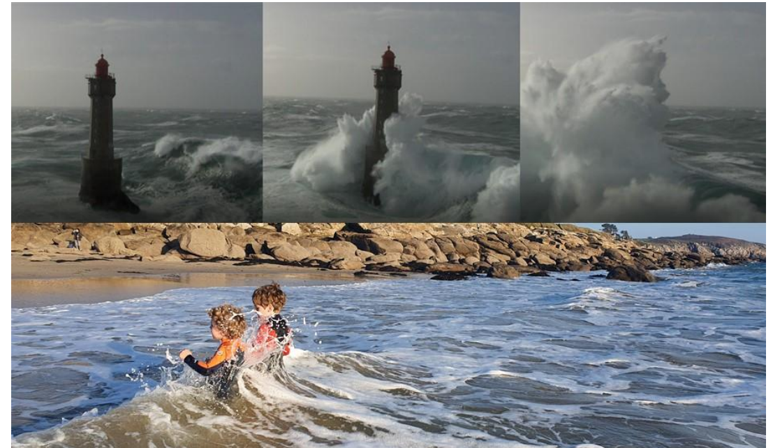
Figure: Top panels : A massive wave slamming La Jument lighthouse. Credit : Air, Vide et Eau. Bottom panel : 2 kids experiencing a slamming load
