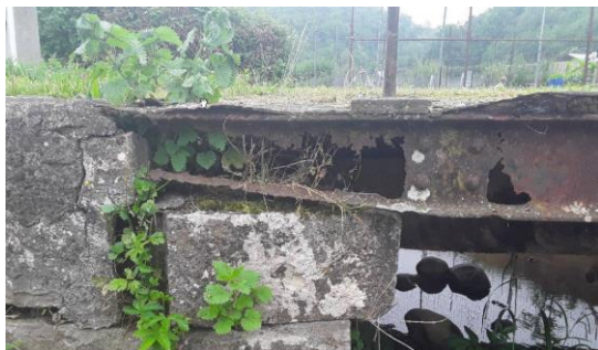
Corrosion perforante
