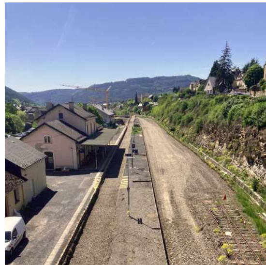
During: with local screened Ballast
