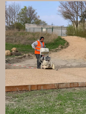
Sciage des joints
