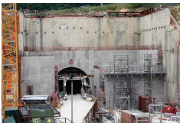
a) Tunnel A86 (site A1)
