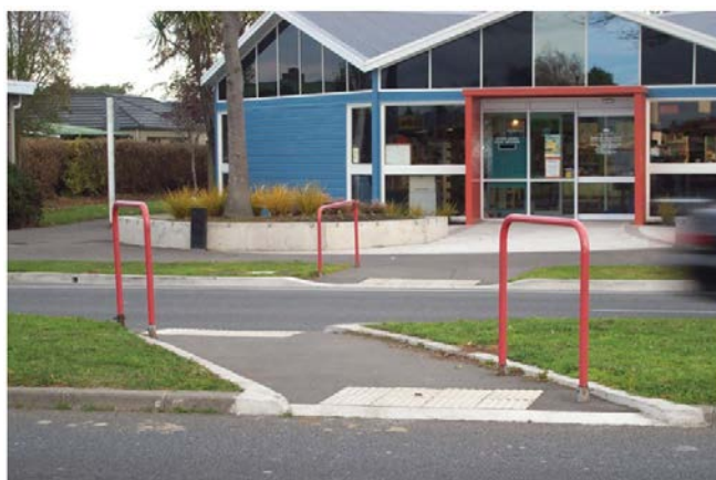
Median with path cut through island, SH 74 Main Nth Rd, Christchurch (Photo: Susan Cambridge)
