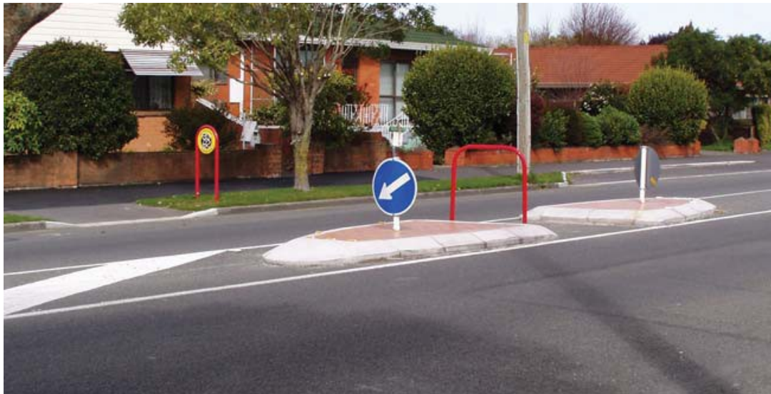
Photo 15.7 – Pedestrian island, Highsted Rd, Christchurch (Photo: Tim Hughes)
