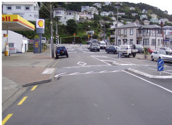
Platform with good footpath to road contrast, Kilbirnie, Wellington (Photo: Tim Hughes)
