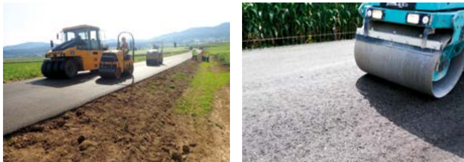
Figure 7 / ORRAP Suisse & France - Compactage. Source Cerema
