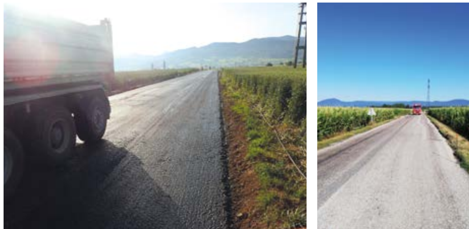
Figure 2 / ORRAP Switzerland & France - Substrate primer/single-layer coating Source Cerema
