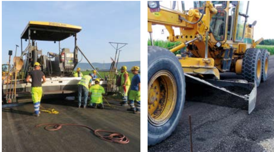
Figure 3 / ORRAP Switzerland & France - Paving with paver/grader Source Empa & Cerema
