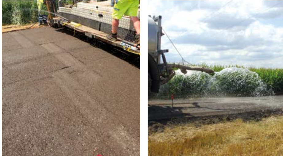
Figure 4 / ORRAP Switzerland & France - Spray watering. Source Cerema
