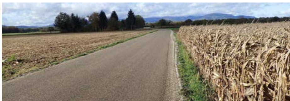
Figure 8 / ORRAP France - Surface dressing for finishing. Source Cerema
