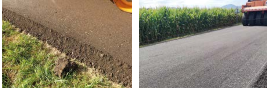
Figure 6 / ORRAP Switzerland & France - Difficult compaction on pavement edges Source Cerema
