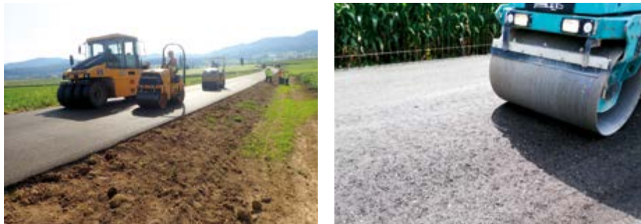
Figure 7 / ORRAP Switzerland & France - Compaction. Source Cerema
