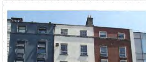
28 Westmoreland Street, Dublin 2
