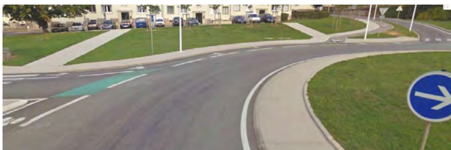
Figure 61 – Hard shoulder in a roundabout
