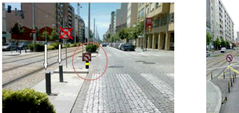
Figure 81 - Porto, Av. da República in Matosinhos, traffic signals and road signs to forbid left turn movements
