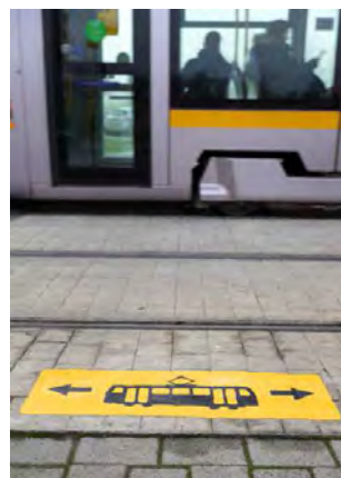
Figure 127 – Dublin, tram warning pavement marking at uncontrolled crossing at Luas Stop
