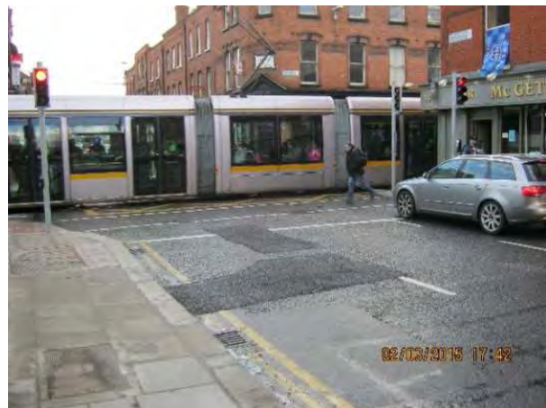
Figure 108 – Dublin, junction after modification
