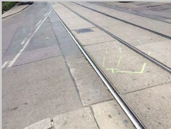
Figure 11 – Example in Vienna – marks made on the carriageway made by the operator [Source: Wiener Linien]
