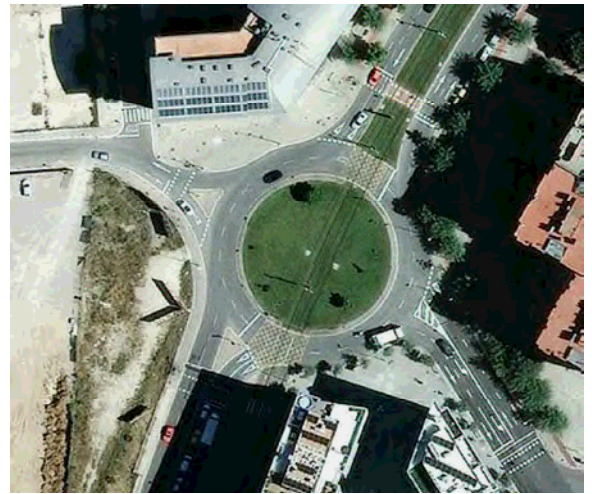
Figure 94 - Barcelona, roundabout (Carretera d'Esplugues - Joan Maragall)
