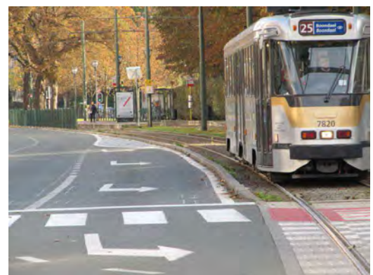
Figure 76 – Brussels, Hansen Soulielaan – Louis Schmidtlaan, creation of an extra lane for left turn
