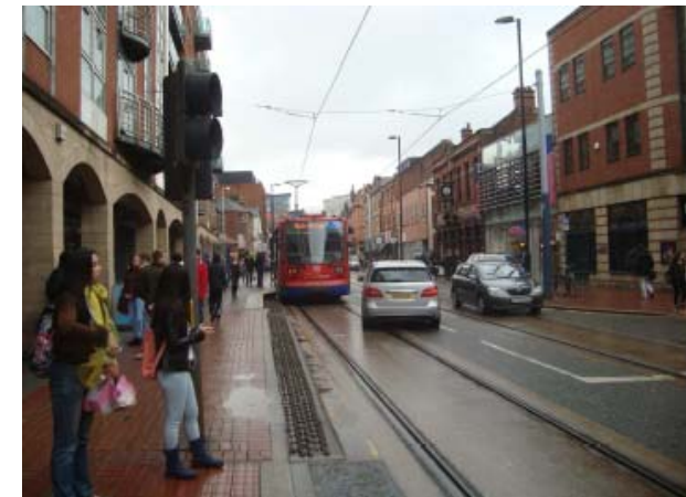
Sheffield: example of configuration with lateral track/ no dedicated platform/ mixed traffic
