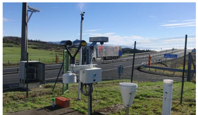
Fig. 3 Fageole highway weather station on the E70 motorway
