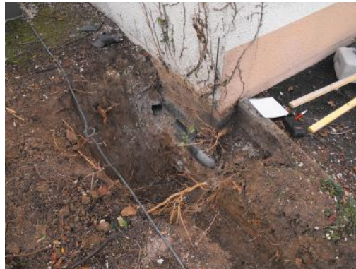
Figure 6: excavator drilling (with numerous roots)
