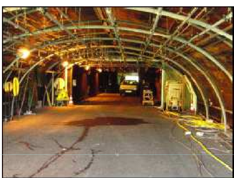
View of the platform track of the Clermont-Ferrand laboratory
