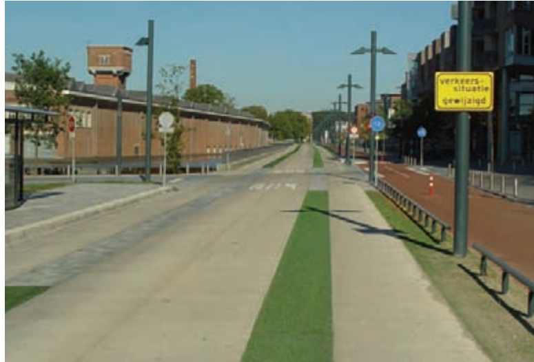
Warning lights on ground at the crossing for the cars, flashing at each bus arrivals. The yellow sign states: "Traffic situation changed"
