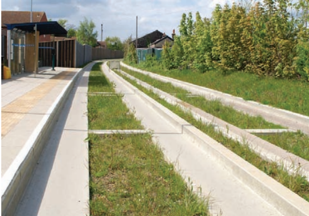
The concrete guided way along a station
