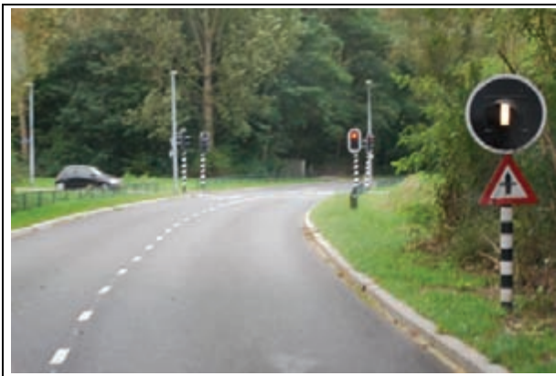
Almere: announcement of the green phase, allowing a limited speed of the buses, at not over 40 km/h, for safety and comfort reasons
