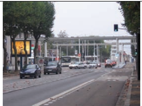
Lorient, type C with service streets on the sides, just before the biggest interchange with the rail station
