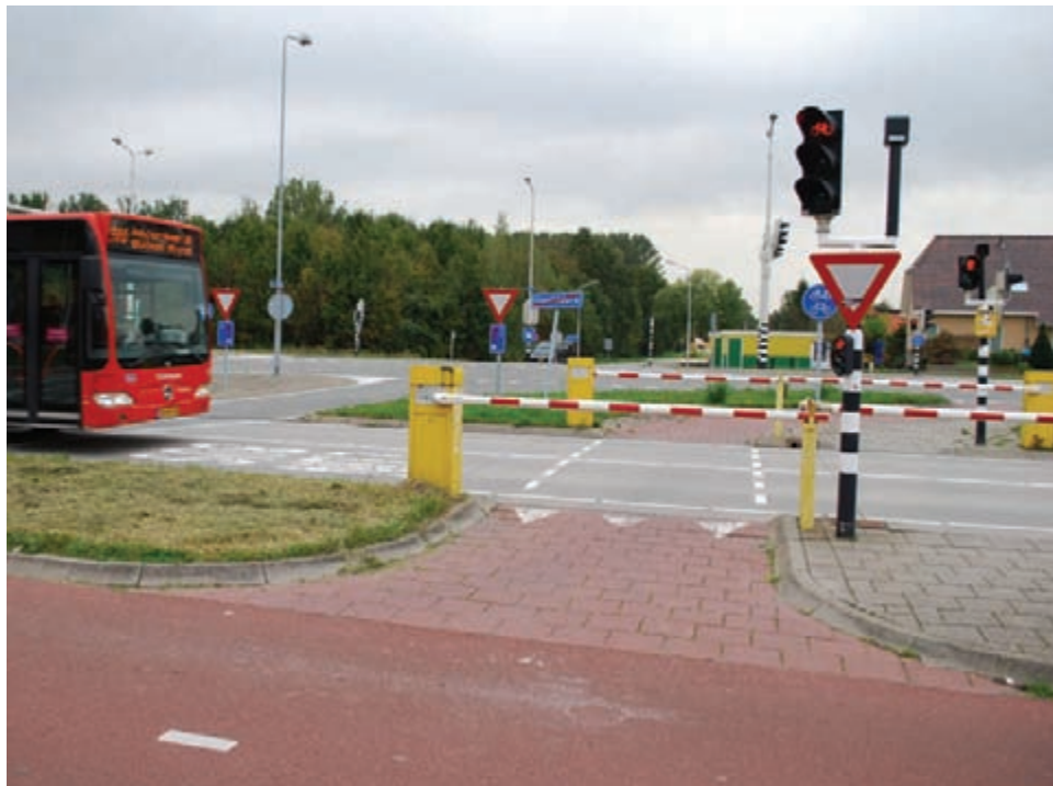
Zuidtangent: crossing with pedestrian and bicycles are protected with barriers and traffic lights along the section that can be over 70 km/h
