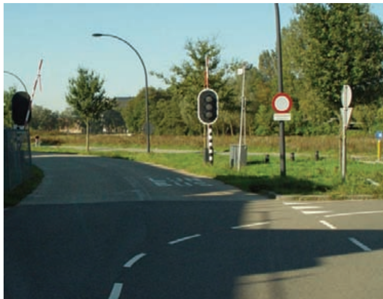
Twente; access control with barriers and traffic lights
