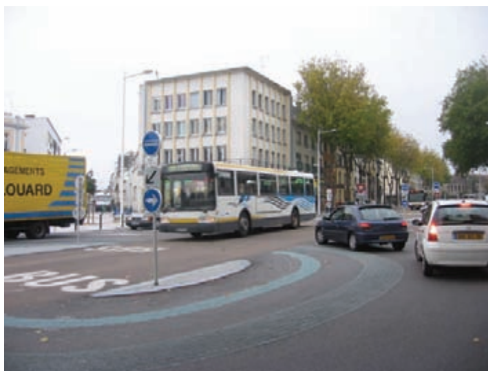
The bus crossing the roundabouts, with a total priority, without traffic lights
