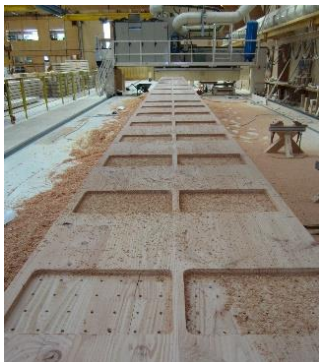
Fig. 21 Reserved spaces dug in beam
