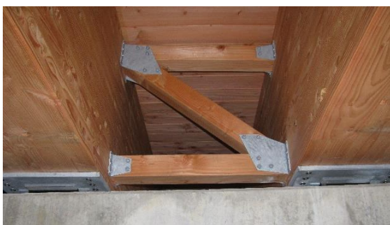
Fig. 26 Bracing on pier
