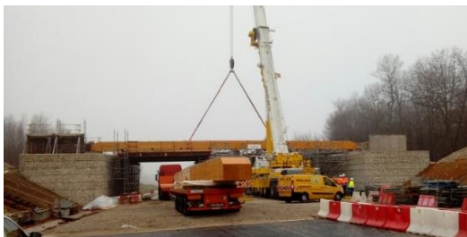
Fig. 31 Beams being put in place with the crane
