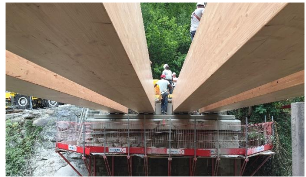
Fig. 20 View of the 4 girders
