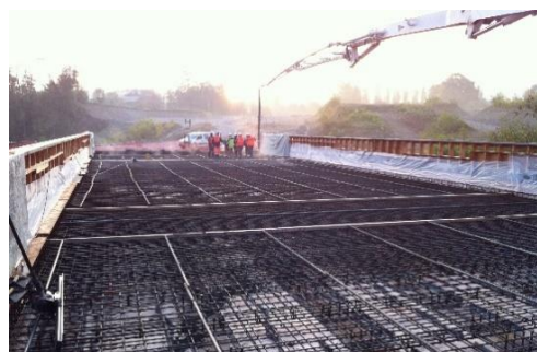
Fig. 27 Casting of the slab
