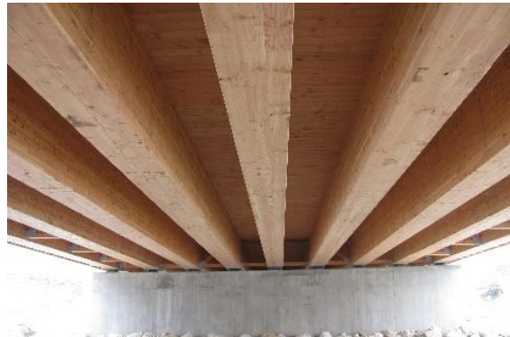
Fig. 24 Intrados view of deck
