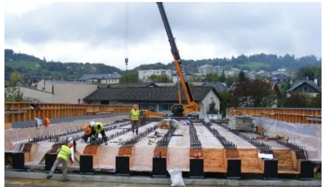
Fig. 25 Beams with metal plates for connection
