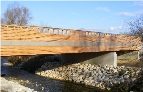
Fig. 23 Lateral view of bridge
