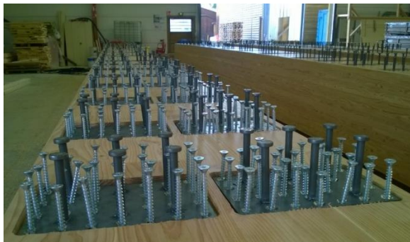
Fig. 8 View of studs welded on steel plate with screws before screwing
