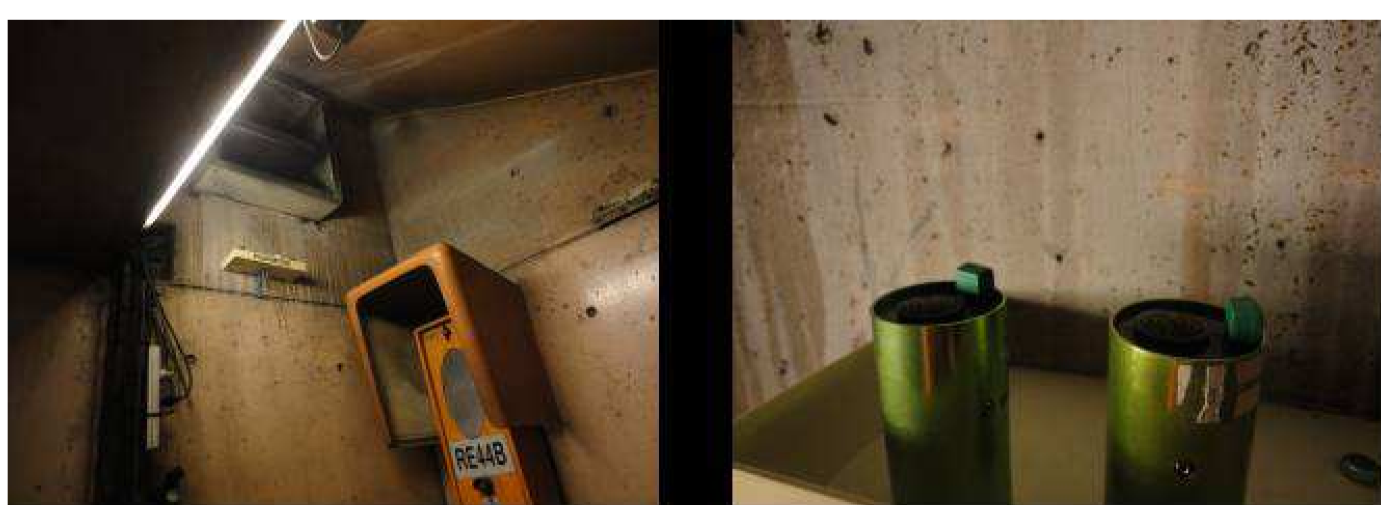
Photo 5 - Installation of the pollution sensors in the Guy Môquet tunnel
