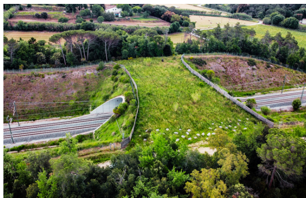
Figure 4: Wildlife passages allow to reduce habitat fragmentation and reinforce green infrastructure (Photo by Minuartia)
