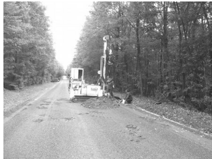
Illustration 33: The probes are installed by the drill
