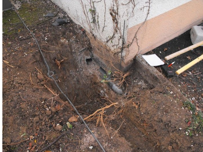
Illustration 47: excavator drilling (with numerous roots)
