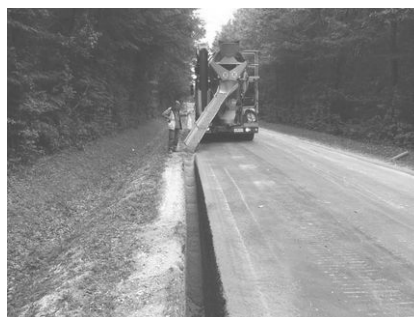
Illustration 30: Pouring concrete by concrete mixers
