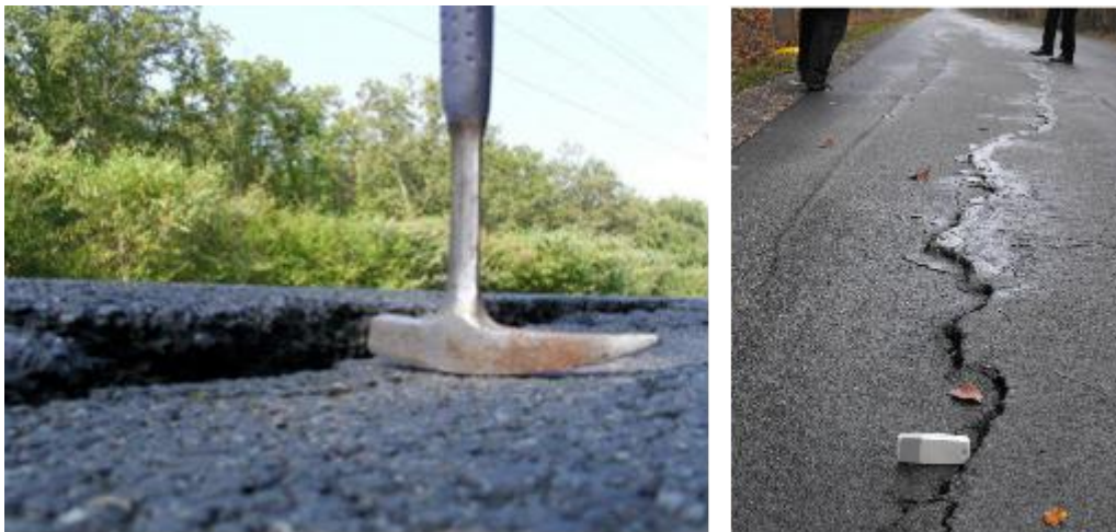
Illustration 25: typical disorders on roads due to drought
