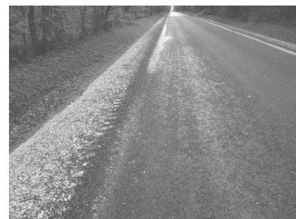
Illustration 31: view of the double surface dressing
