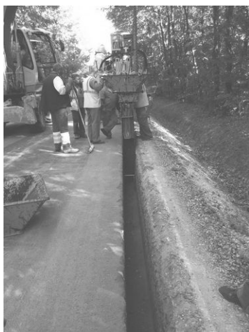
Illustration 29: excavation using a trench excavator
