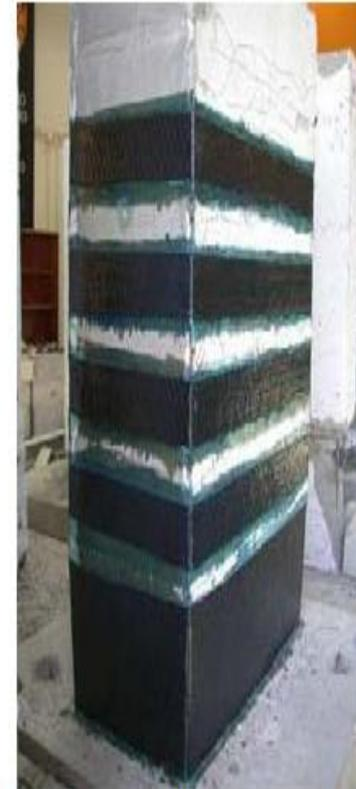
Figure 3. Hollow piers before and after the shear retrofitting with 2 layers of CFRP strips (UP).
