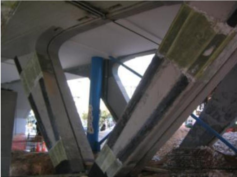
Strengthening of 108 bridge piers with Tyfo UC Strips and Tyfo SEH-51A.
