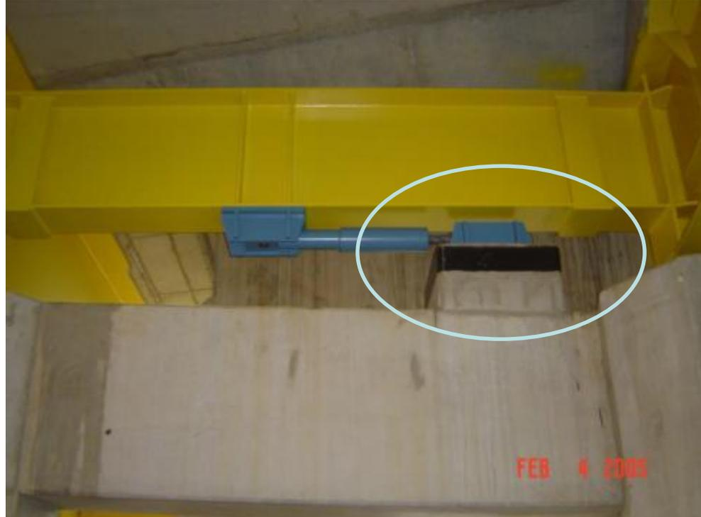
Strengthening of 28 seismic absorbers' shear-keys with Tyfo SCH-11UP.
