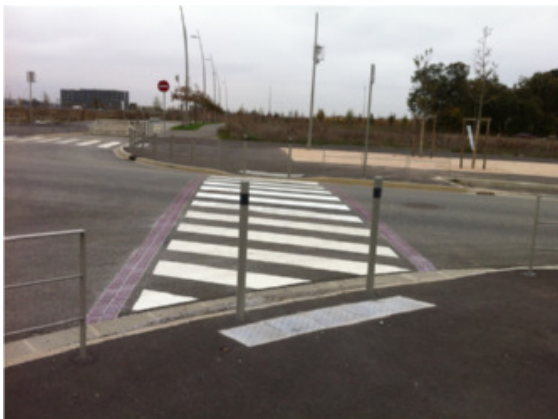
Crossing marked out by contrasting glued strips of paving in Toulouse
