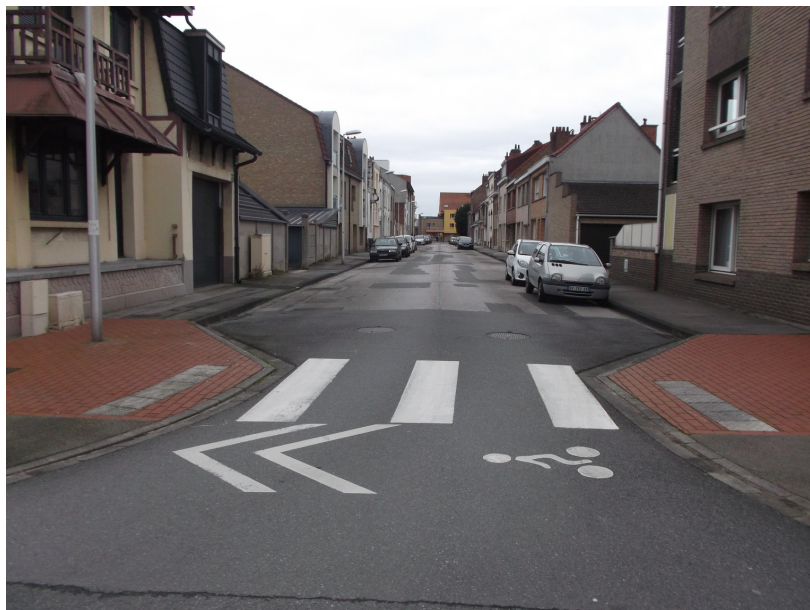
Example of junction design with curb extensions in Dunkirk Credit: Communauté urbaine de Dunkerque
