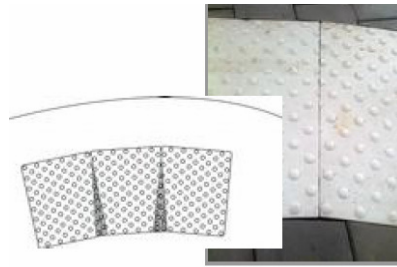
Rounded pavement with fitted warning surfaces in Lille
